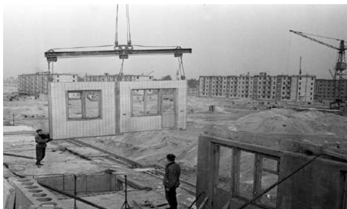
Fig.3 – Prefabricated panel construction. Source: TsDKFFA of Ukraine
