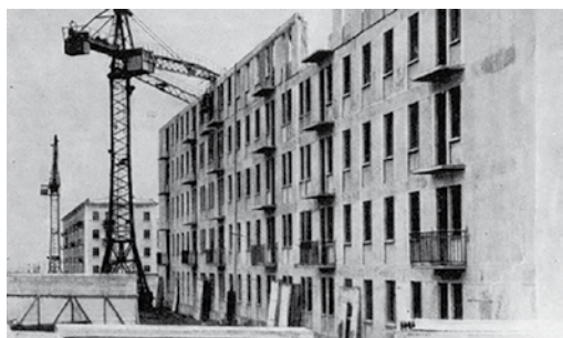
Fig. 2 – Large-block housing construction. Source: Retro View of Mankind's Habitat
