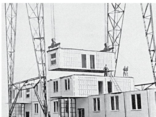
Fig. 4 – Mounting volumetric blocks. Source: Ataev. 1967. Technology and Economics of Volume-Block House Construction
