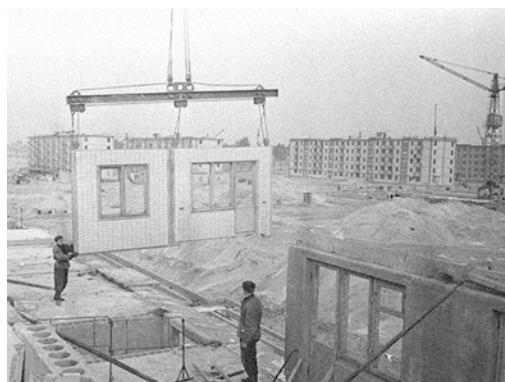
Fig. 3 – Prefabricated panel construction. Source: TsDKFFA of Ukraine
