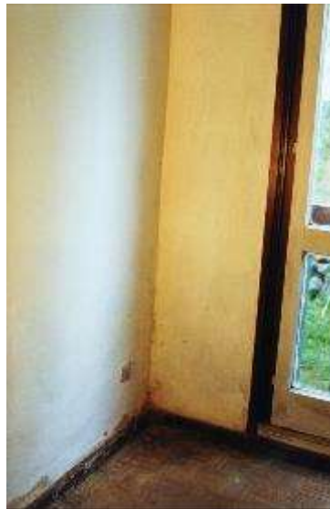
Figure 61. QM: Interior humidity coming from exterior panels, caused by the incorrect assembly of the panels or by the lack of compression in the sealants of the panels' joints
