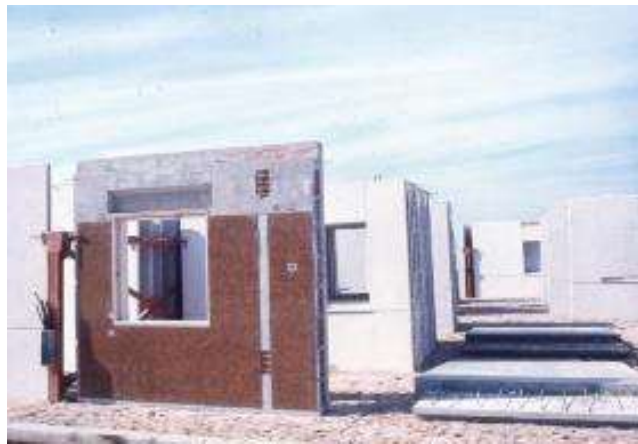
Figure 31. Storage area of the exterior panels and prefabricated elements (interior panels) storage yard
