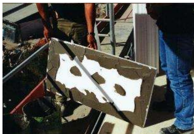
Figure 65. Building work in progress (Science Faculty of Lisbon Building) – The insulation board with adhesive coat applied with points and bands
