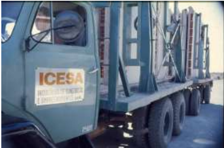
Figure 33 - Transport of vertical panels
