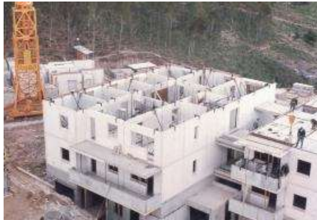
Figure 43. Assembly of the panels on site
