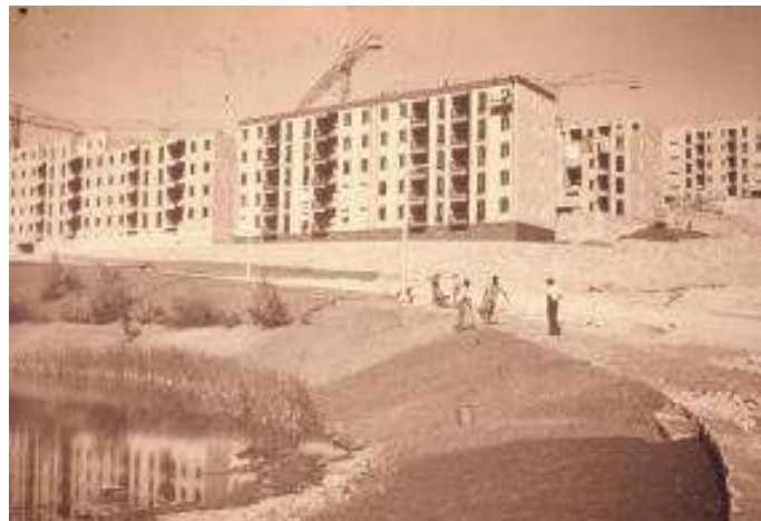
Figure 46. Assembly of the heavy panels on site and view of the first completed buildings
