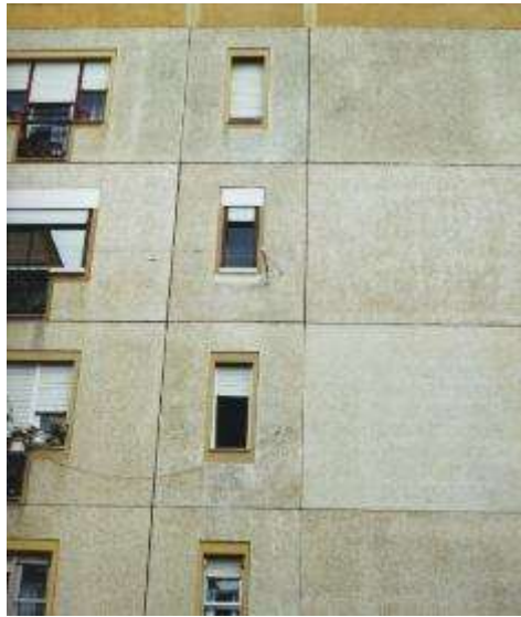
Figure 60. SAC: Micro-fissures in exterior panels
