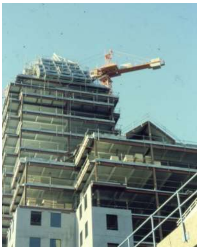
Figure 2. Partial prefabrication of exterior walls – conventional metallic structure
