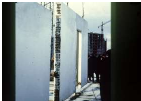
Figure 45. Assembly of panels on site
