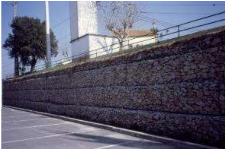
Figure 52. Gabion retaining wall
